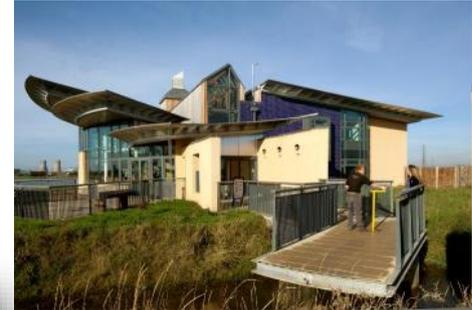
oversailing south facing roofs provide solar shading in the summer but allow solar gains in the winter
