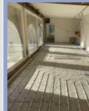
Underfloor heating installation at Sandhoe
