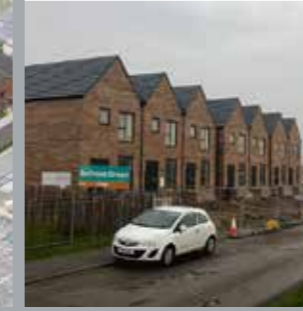
Construction underway at Silksworth
