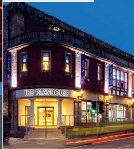
Alnwick Playhouse has reopened after a £3.3m refurbishment.
