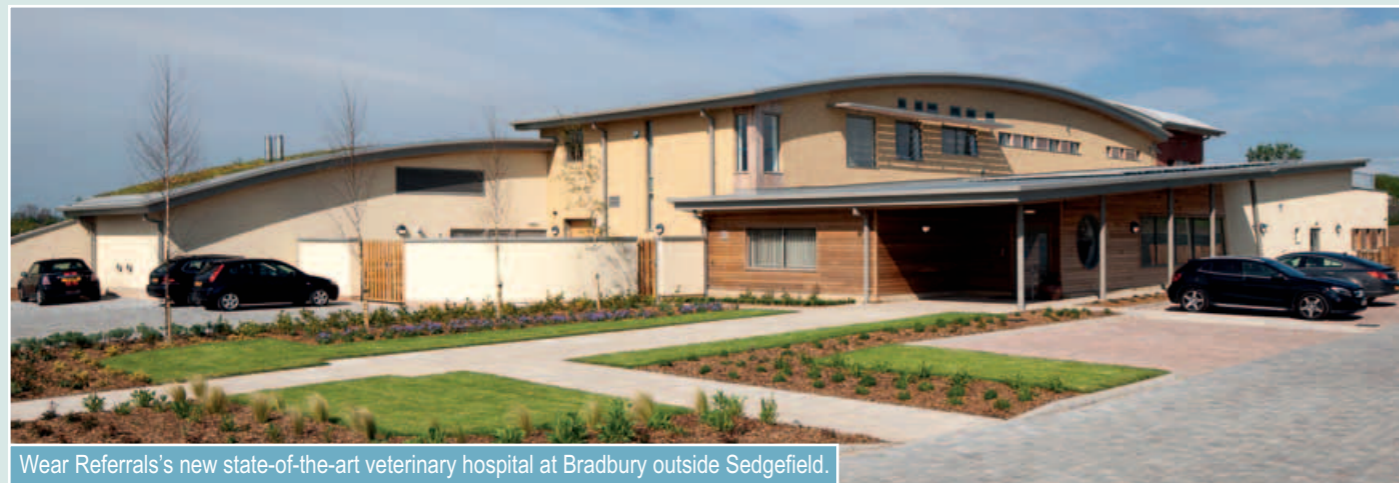
Bright and airy front-of-house facilities for anxious pet owners.
