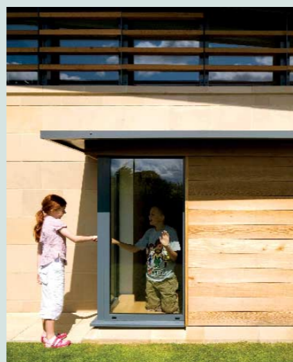
Sure Start Children's Outreach Centre at Barnard Castle features these 'creeps' for small children which jut out of the building like mini bay windows.
